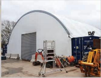
The benefits of using a Zappshelter end wall include additional weather protection from driven rain and snow in exposed areas. When working with sensitive equipment or materials, or when applying coatings such as paint or lacquer, it is essential to keep the area dry. The use of end walls also means some heat may be retained.
